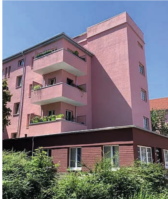
IR-reflective façade paints help reduce the heating of building surfaces.
